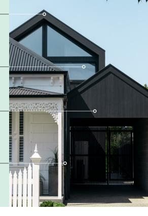
'The new wall needed to align with the existing hallway, so we were restricted in wall thickness. We were able to align the old and the new by using Axon™ Cladding, which is much narrower than a brick or block wall.'
